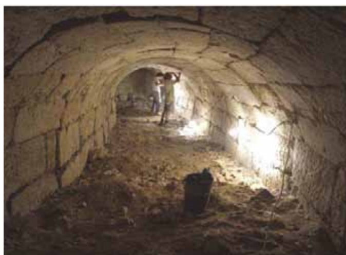
Vaulted corridor at the base of the fortress
