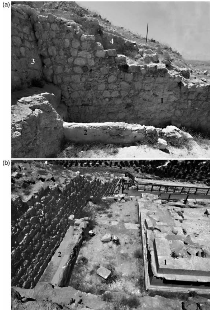
Fig. 7. View of the later stairway built over the irrigation basin of the mausoleum. (a) Looking west: (1) later stairway; (2) irrigation basin; (3) southern wall of the burial lot; (4) earlier stairway (B. Arubas). (b) (1) mausoleum podium; (2) irrigation basin; (3) later stairway (J. Patrich).
