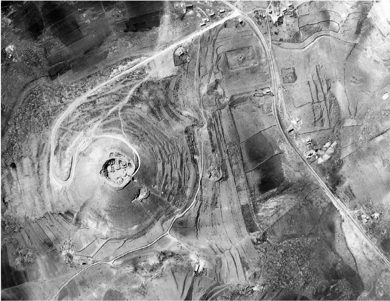
III. A.13. Aerial photograph of Herodium and its surroundings, taken in 1967 (approximate scale — 1:7,000).
